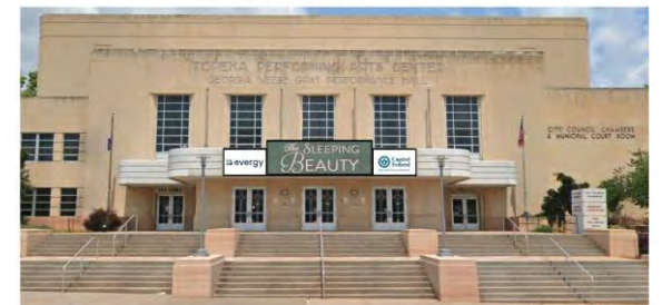
Daytime View - Marquee
