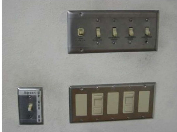
Typical large classroom lighting controls are mostly original. Dimmers are not suitable for fluorescent lamp dimming.
