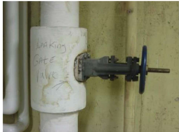
Main steam shut-off valve indicated to leak. Leaking steam a safety hazard due to high pressure/temperature steam.
