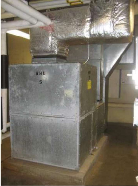
Cooling-only VAV AHU-5. Original dual deck unit replaced to serve VAV box zones.
