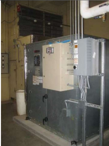
AHU-1 fan has been replaced and VFD provided.
