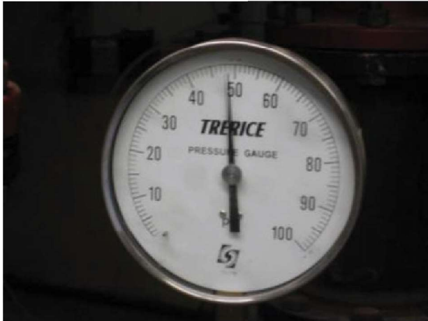
Cooling tower pump pressure gauge (upstream of 30 valve) 49 PSI of pump pressure is required to pump from basement to rooftop tower. Very energy intensive. Redundant pumps are 30 HP each.
