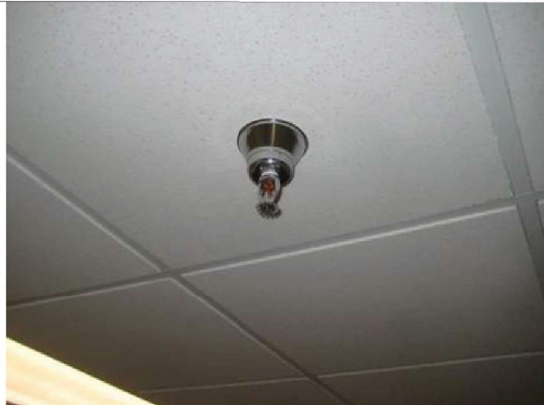
Typical “newer” basement sprinkler head located in past basement renovation areas. Only basement is sprinkled.
