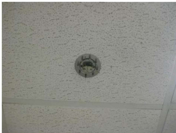
At basement, all original fused link type sprinkler heads need replacement with modern quick-response heads.
