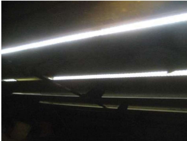
AHU-6 outside air dampers lack edge seals, don't provide full closure and waste energy.
