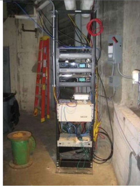
KTWU transmitter rack is located exposed in penthouse mechanical room. Additional protection is recommended.
