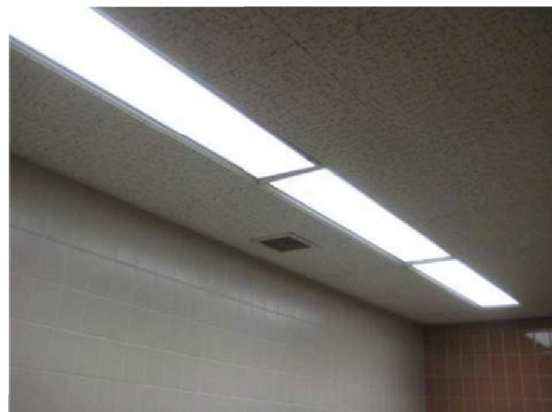
Typical small exhaust grille at restrooms. Restroom exhaust in general is inadequate.
