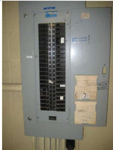
Typical original branch panelboard. Parts no longer made. Panels full. Replacement recommended.
