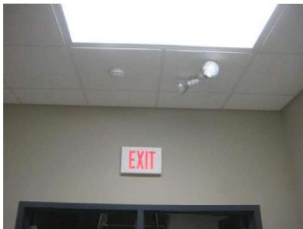
Typical surface emergency lighting screw-in lamp holder/fixture. Overall emergency lighting coverage is fair. A mock power outage is recommended to determine actual performance and identify areas needing improvement.
