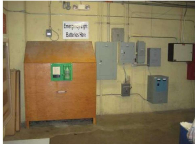
Lead-acid battery system with emergency lighting inverter on wall at right serves all egress lighting in building.
