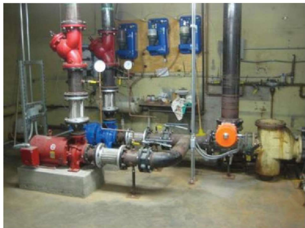
Cooling tower / condenser water pumps. Single basket strainer requires system shutdown to clean. Lack of automatic filtration system requires regular manual cleaning and flushing of strainers.
