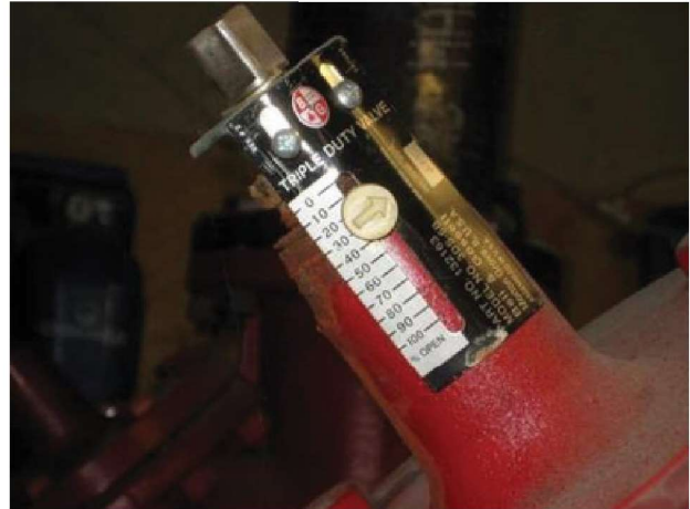
Cooling tower pump 3D valves are 72% restricted to limit flow. Very wasteful parasitic energy loss. VFDs recommended.
