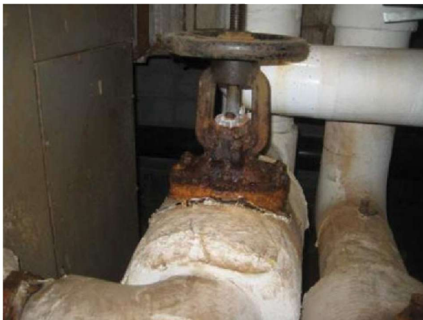
Typical OS&Y gate isolation valves at AHUs are rusted and need replacement with ball valves or butterfly valves.
