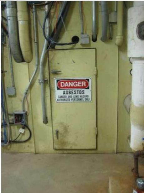
Asbestos indicated at tunnel systems. Appears most building piping systems have been abated.
