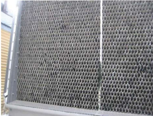
Cooling tower fill needs replacement. Chemical treatment needs adjustment to lessen scale.
