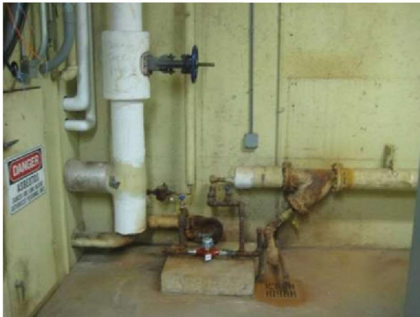
Campus steam supply and condensate return at tunnel. Traps, strainers and valves should be replaced. Long term replacement with gas heating system is recommended.
