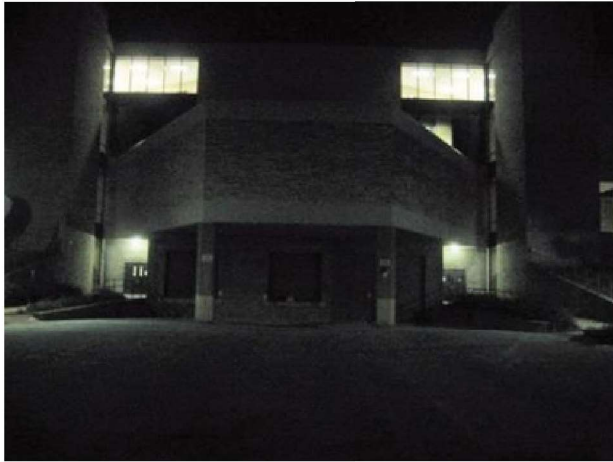
South façade, loading dock and parking lighting.
