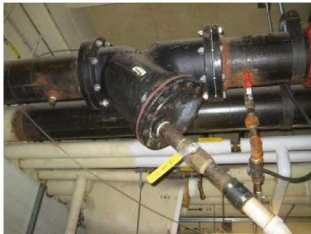
Tower return strainer is leaking, needs repair and new seals. Steel tower piping should be checked for excessive pitting and erosion especially at bottom of vertical drop from penthouse.
