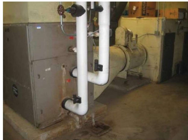
Original built-up AHU-4. Single zone with hot/cold deck mixing. Overall condition poor to fair.
