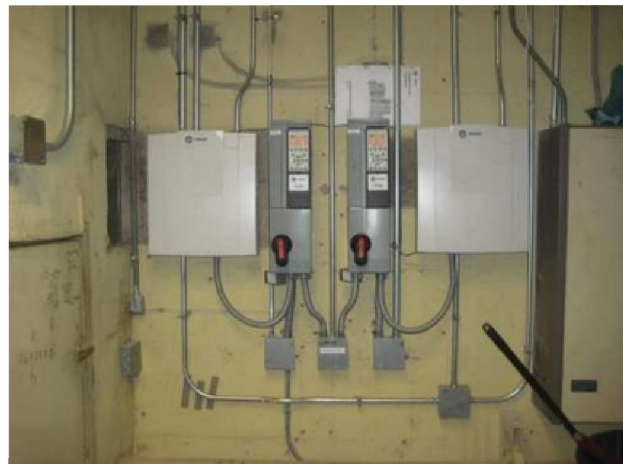
New AHU-3 and AHU-4 VFDs. At fans original inlet vanes are in fixed position.
