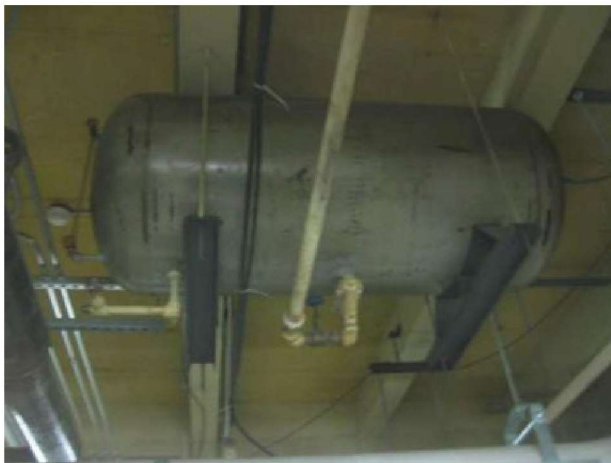
Original HW system expansion tank at structure needs replacement. Old technology tank lacks bladder for air separation and pressure control. New tank would be at floor for ready inspection and maintenance.
