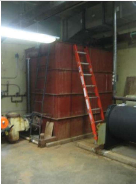
Original remote cooling tower basin is rusted and needs replacement. Removal and use of tower sump is recommended.
