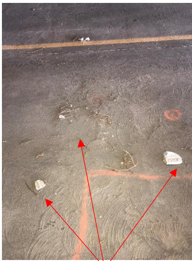
Debris on floor falling deteriorated concrete area above
