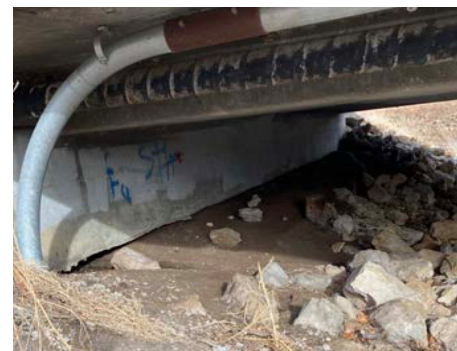
North Bridge Abutment Scour - SW MacVicar Avenue over Ward-Martin Creek
