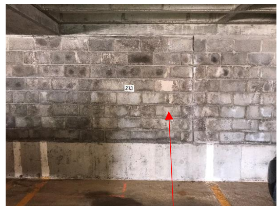
Moisture stains on the inside face of wall of failed elastomeric coating
