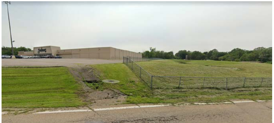
View looking southwest from SW Fillmore St with stormwater detention basin and berm in lower right. (May 2019)
