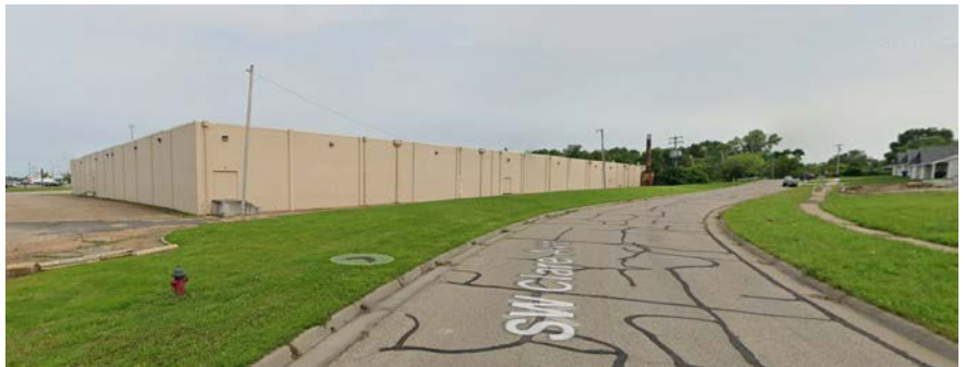
View looking southeast from SW Clare Ave. Recently built duplexes on the right. (May 2019)
