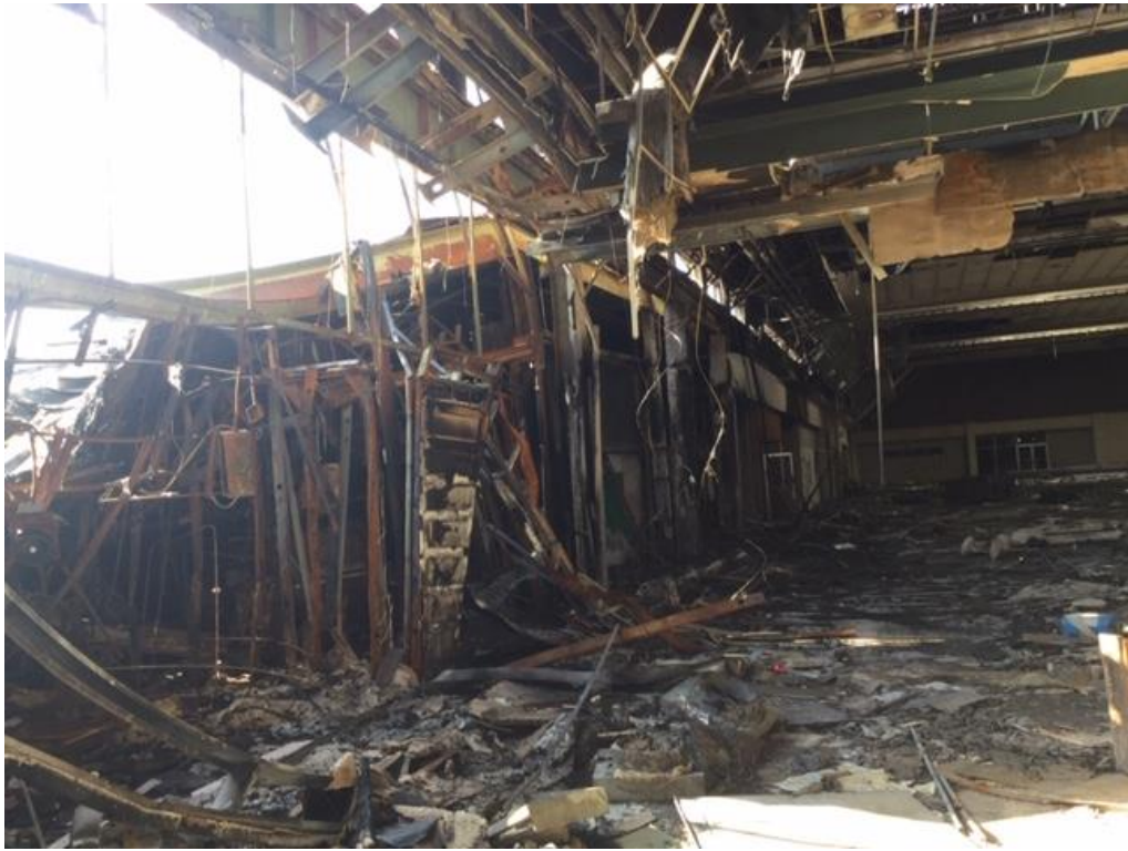
Roof destroyed by fire debris all over floor load bearing walls compromised
