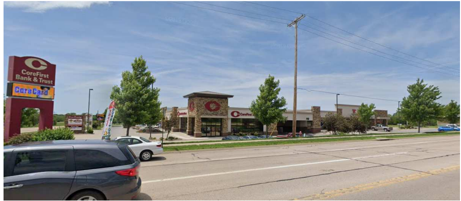
Subject Property – View from Croco Road East of Property
