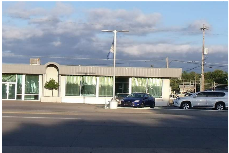
From west side of SW Topeka Boulevard facing front of subject property at 1834 SW Topeka Blvd.
