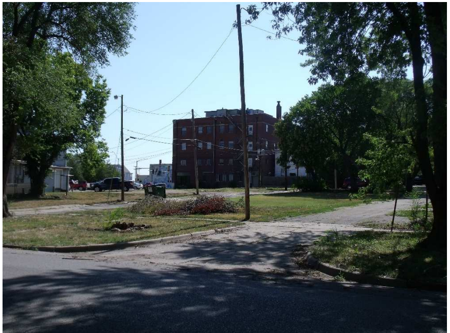
Facing northeast from west side of SW Tyler Street with view of vacant property proposed for new building with 8 residential units (Area C), with existing driveway on right and public alleyway on left, and The Casson Building in background
