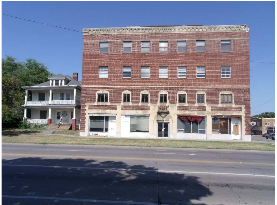
Facing west from east side of SW Topeka Blvd with view of front facade of The Casson Building proposed for reuse for 23 residential units, with adjacent multi-family residential structure on left
