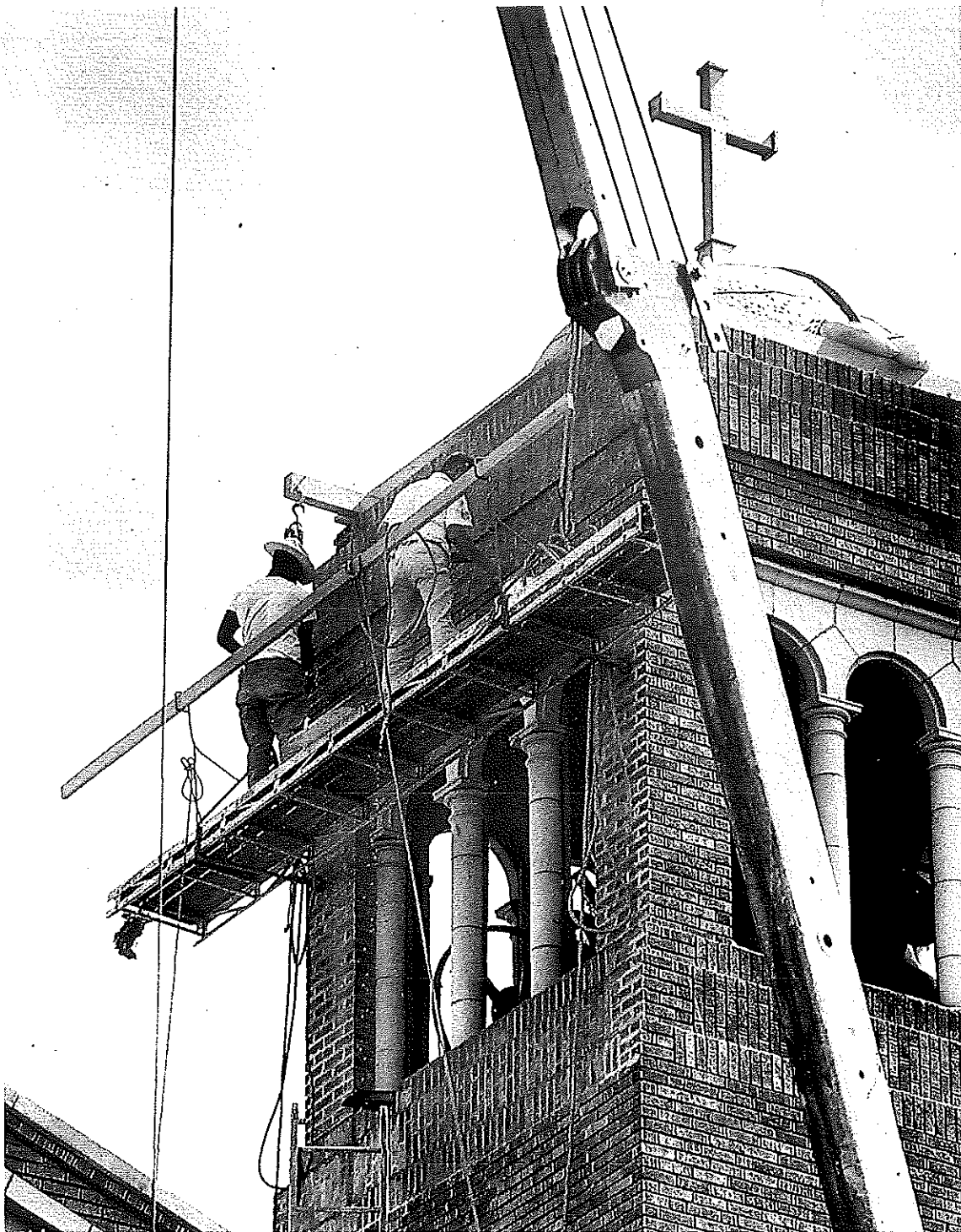
ched precariously above S.W. 8th Avenue, two workmen replace bricks in the east bell tower of Assumption Catholic Church. Bricks and tiles were ripped from the tower by the tornado.
