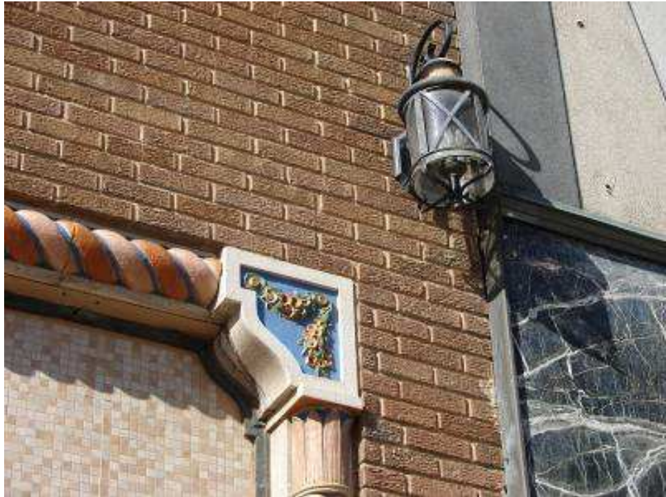
Detail of a commercial building in Downtown Topeka.
