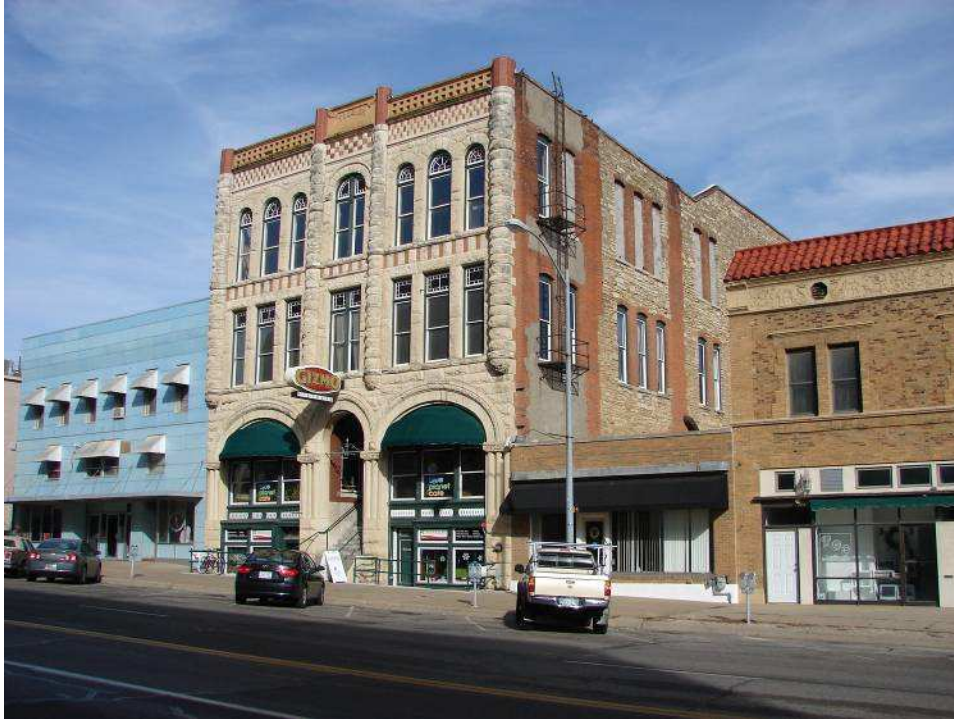
Privately rehabilitated commercial building in Downtown Topeka.
