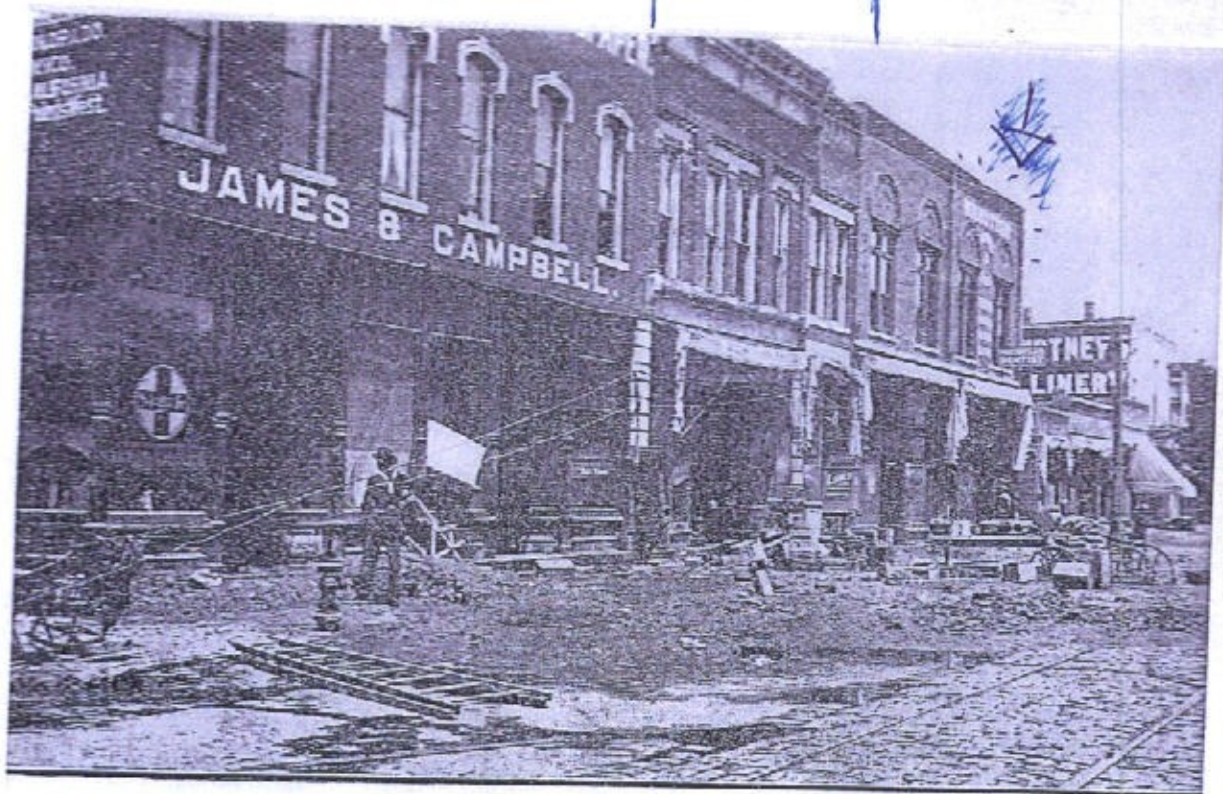
ON KANSAS AVENUE, NORTH TOPEKA, AFTER THE FLOOD.
