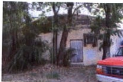
903 N Kansas Ave. West elevation. Finch. 10/06/11.
