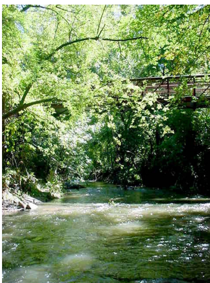
Foot bridge over Shunganunga Creek – Crestview Park
