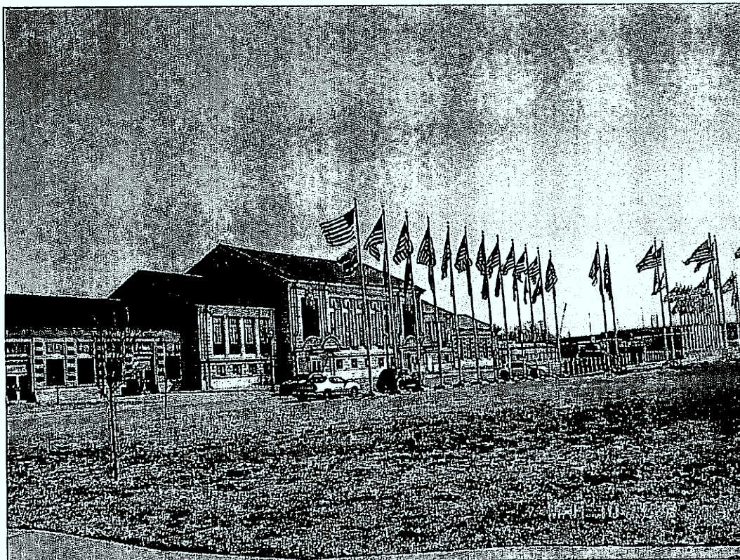
Union Pacific Station – Now Overland Station
