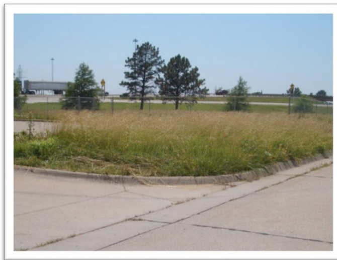
SW 39 th Street cul-du-sac lacks access.
