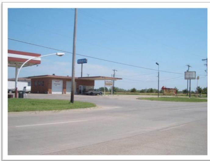
Closed service station on SW Topeka Boulevard reflecting economic obsolescence.
