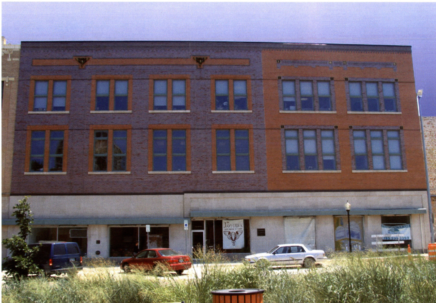
Front (West side)
