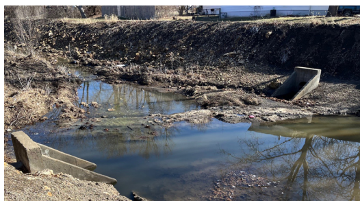
Site B in Washburn Park showing exposed culvert headwalls and displaced riprap at sanitary crossing
