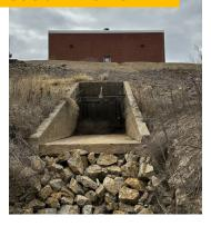
**Outfall D10-26472** has severe erosion at the end of the outfall, and it is unclear if the concrete toe of the outfall is undermined. The repair could include outfall armoring, repairing concrete toe, and consideration of outfall energy dissipation, such as a riprap plunge pool or hardened concrete structures.
