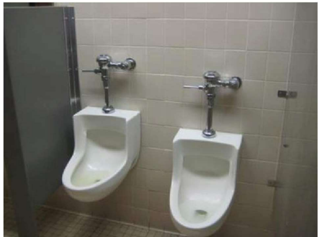
Typical manual urinal flush controls.
