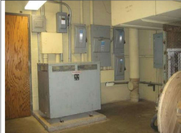
Original east 120/208V distribution equipment uses a feeder gutter and grouping of disconnect switches to serve building loads in lieu of a distribution panel. Transformer efficiency poor compared to new transformers. West 120/208V system is similar.
