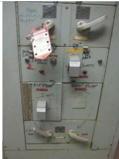
Motor starter "cans" no longer used for starters. MCC parts and switches no longer made.
