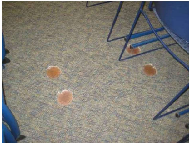
Many floor boxes are no longer used and have been deactivated.
