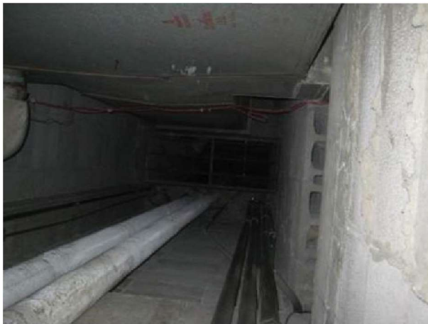
North return air shaft is also open to all floors.
