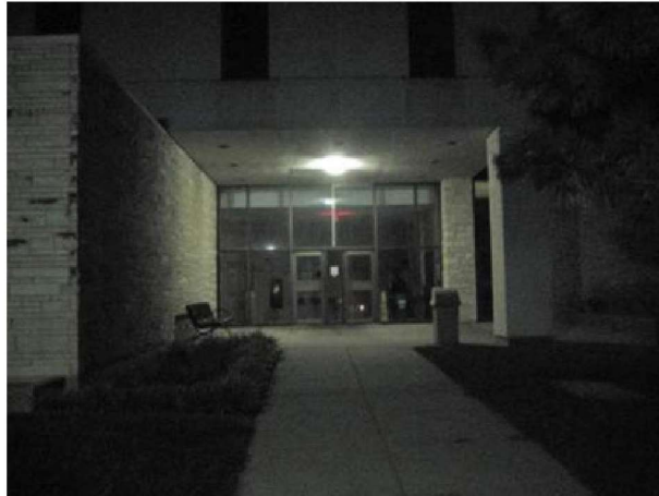
Lighting at the four main entrances is poor and needs improvement suitable for a university environment and student entrances.
