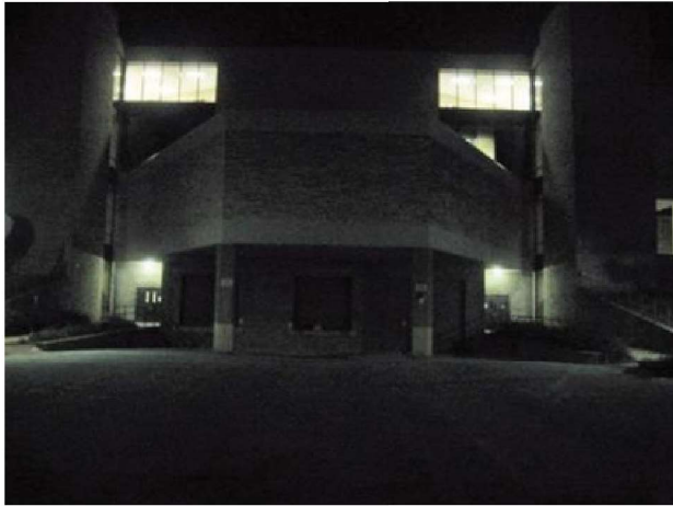
South façade, loading dock and parking lighting.
