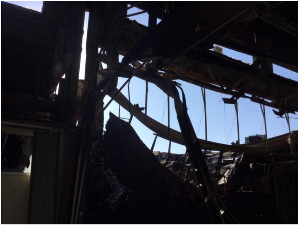
Roof destroyed by fire collapsed inside building
