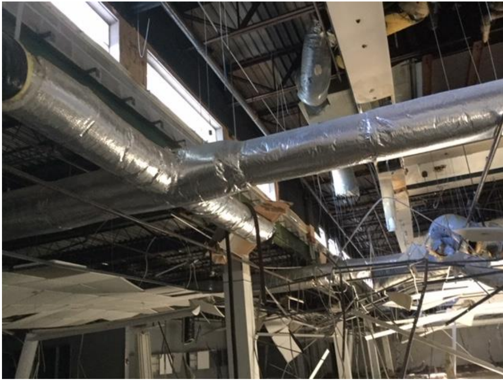
Dismantled ventilation duct, dangling ceiling supports
