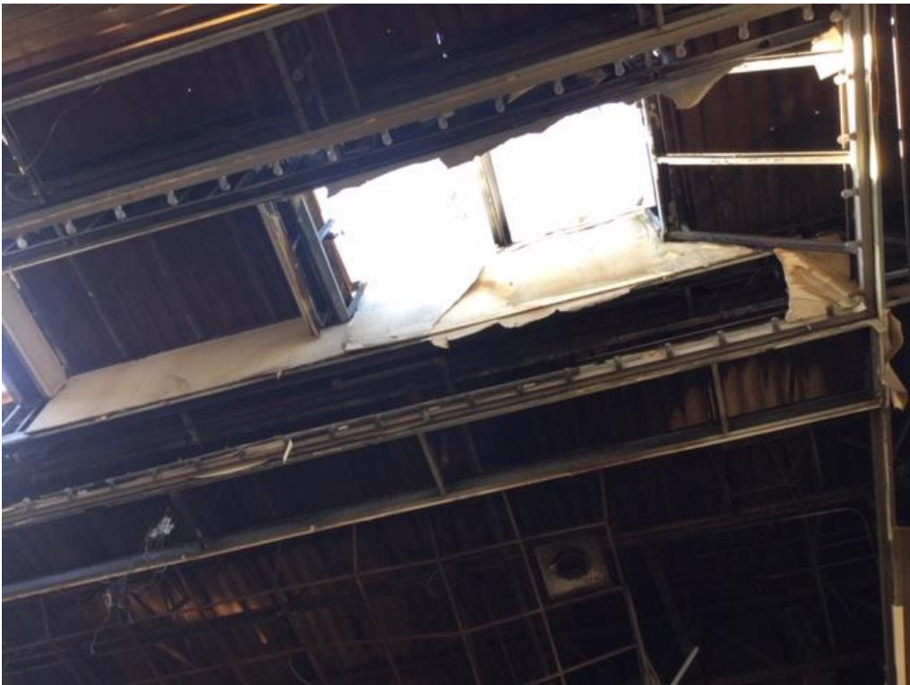
Windows broken out ceiling tile removed ceiling support structure destroyed.
