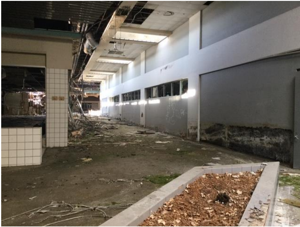
Debris on floor, dangling ceiling supports, and mold on walls
