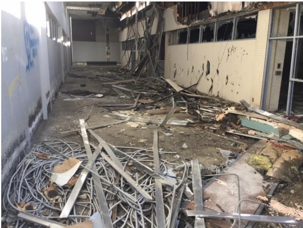
Debris all over floor ceiling supports dangling from ceiling holes in walls
