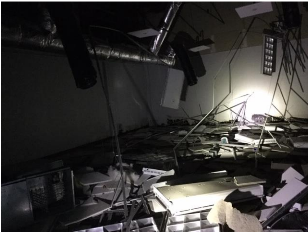
Dangling duct system dangling light fixture dangling ceiling supports floor covered with debris
