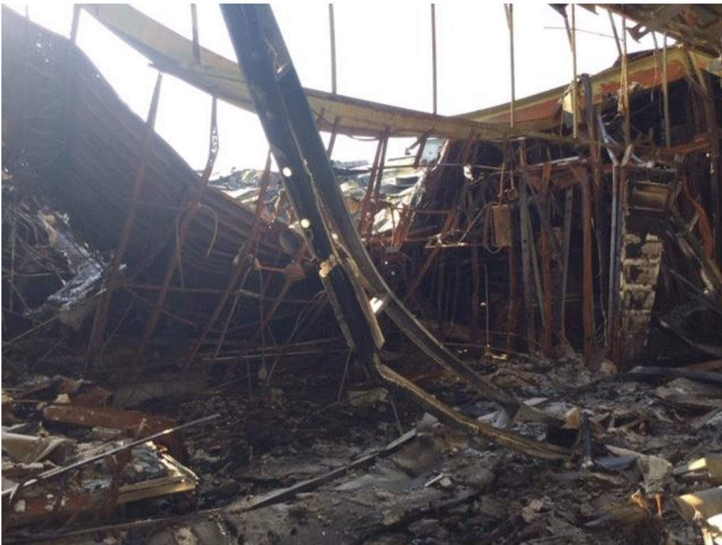
Roof supports collapsed load bearing walls collapsed
