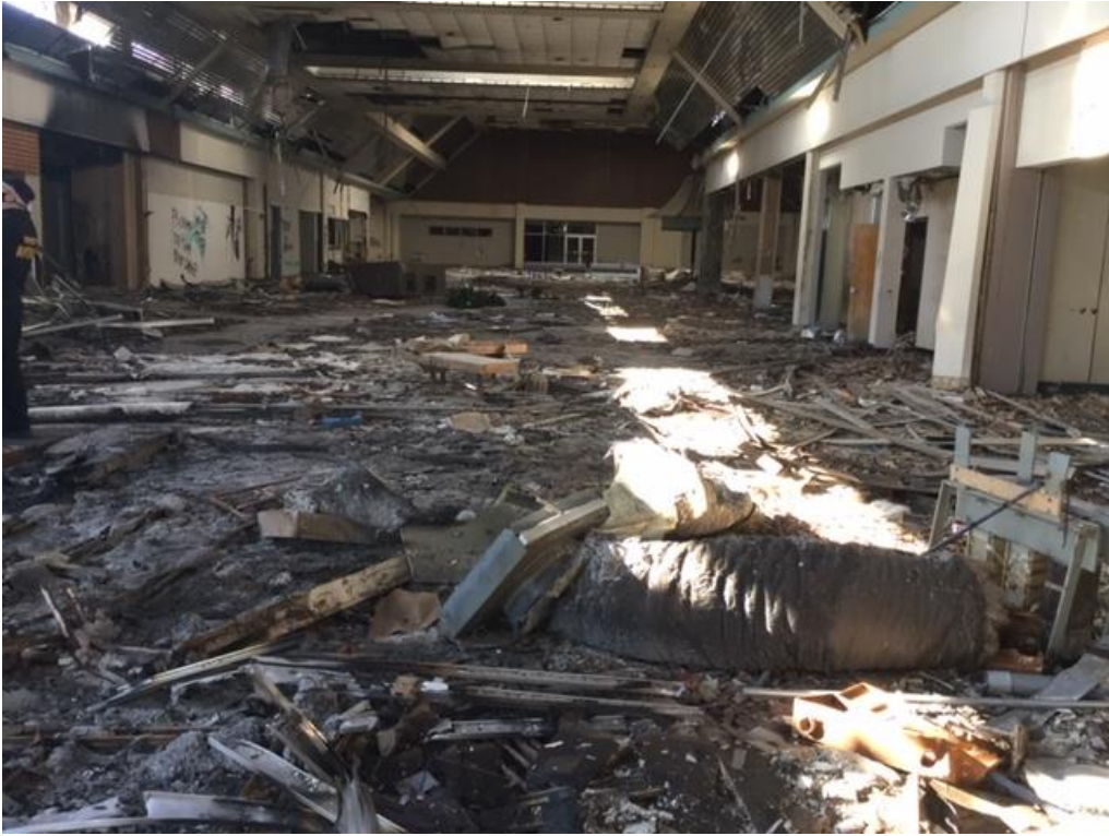
Debris all over the floor ceiling tiles missing windows broken out
