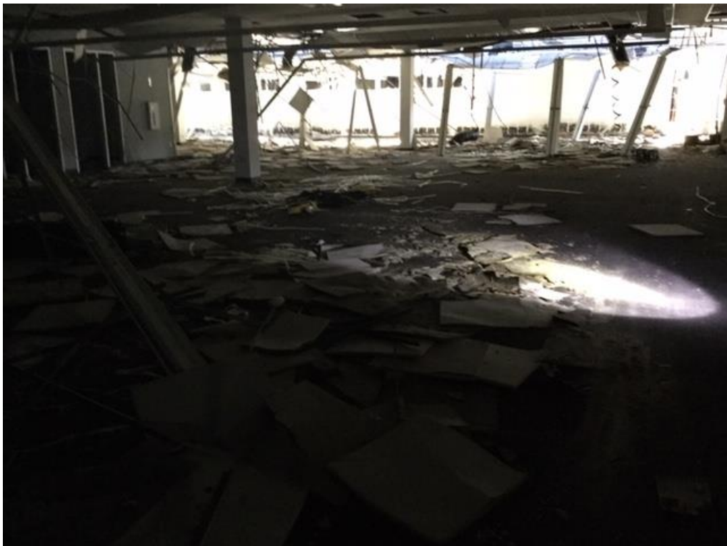
No light debris spread out over the floor ceiling support dangling
