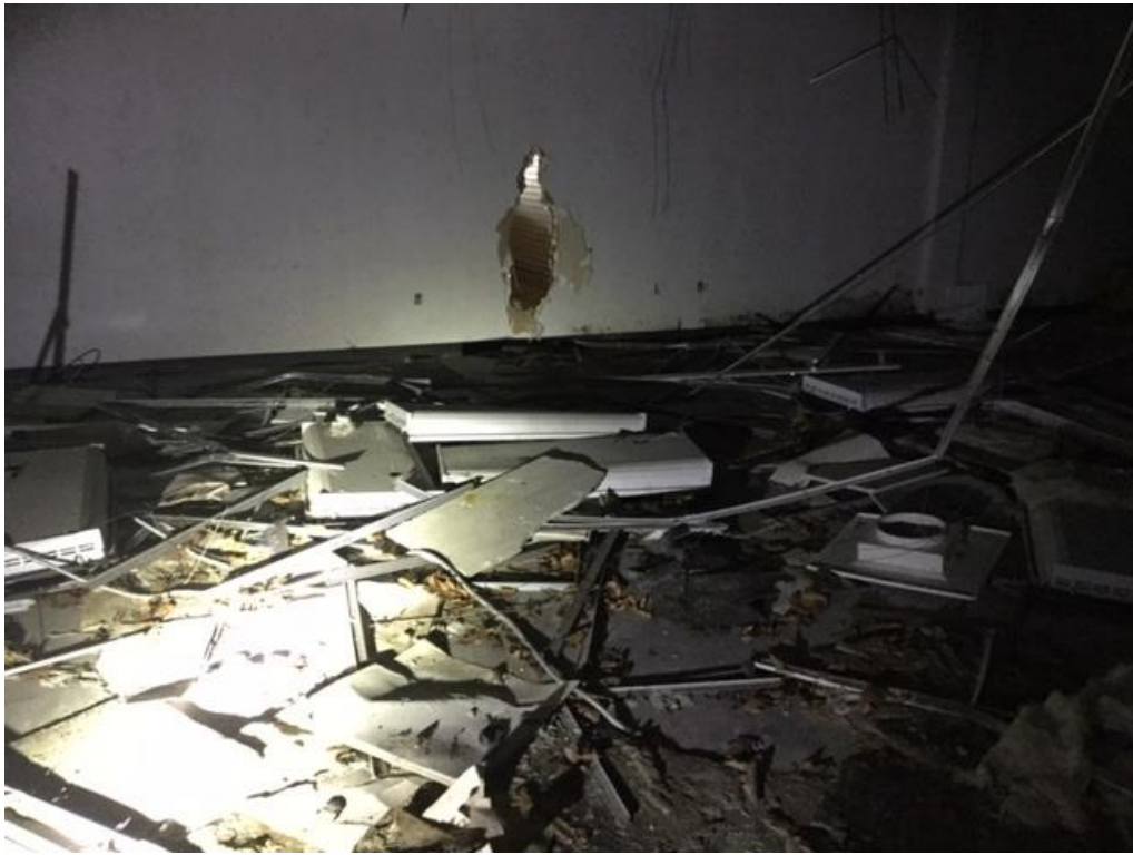
Debris all around hole in wall ceiling supports dangling
